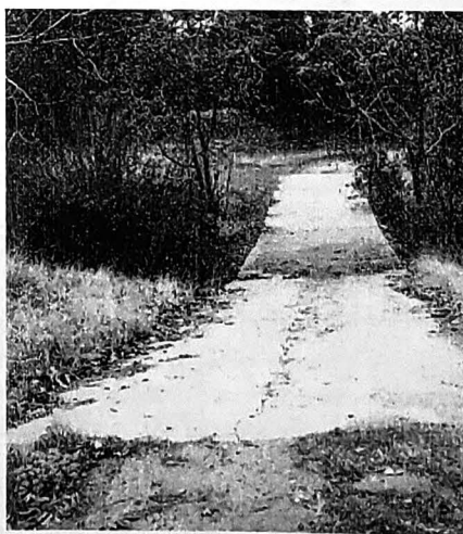
Picture 1-8, Clear Creek Bridge
