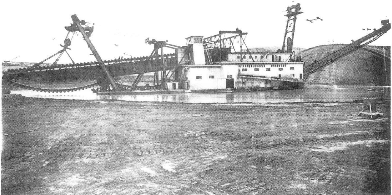
Yuba No. 20, Hammonton, California. Owned by Yuba Consolidated Gold Fields. Digs 175 Ft. Below Ground Level Using 18 Cu. Ft. Buckets.
